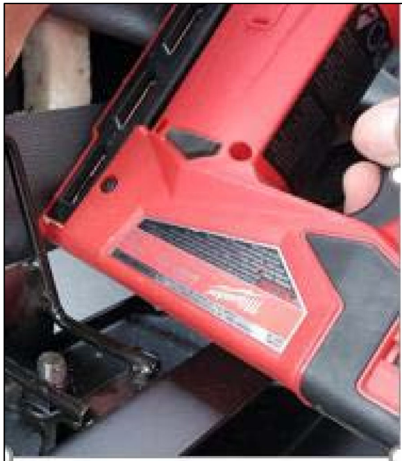
Figure 11: Staple Back of Vinyl Seat Cover onto the Wood Strip
