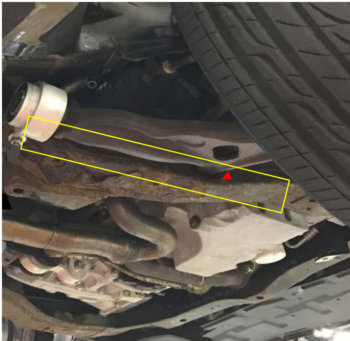
Side View: Non-Damaged Cross member
