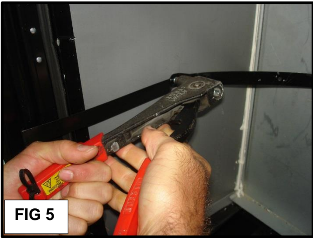
Fig 5: Install each new strap from the kit, with pop rivet gun and 3 rivets from the kit.
