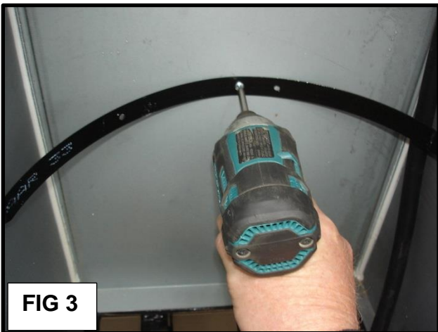
Fig 3: Remove 3 bolts securing the strap with the screw gun and square bit. Pull on the strap to keep tension on the bolts as you loosen them. The nuts will fall off the back side.
