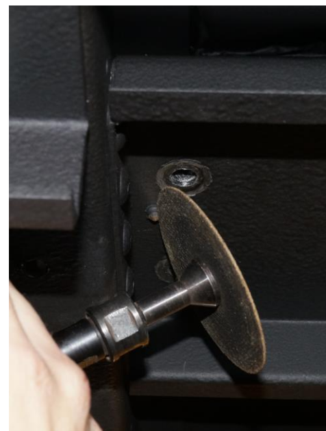
Figure 8 - Cutting rivet with cutting wheel
