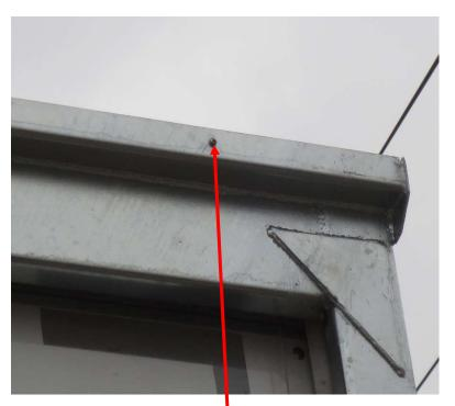
Notice the presence of the Tether Bolt going through the upper rear header indicating that the repair is not needed.
