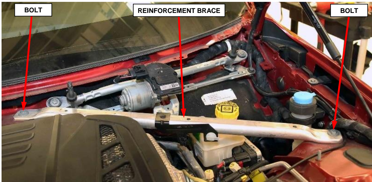
Figure 11 – Left Reinforcement Brace
