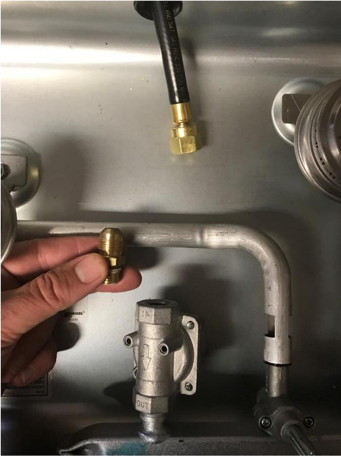
With an adjustable or open ended crescent wrench, disconnect the flex line from the flared coupler, as well as the coupler from the cooktop manifold.
