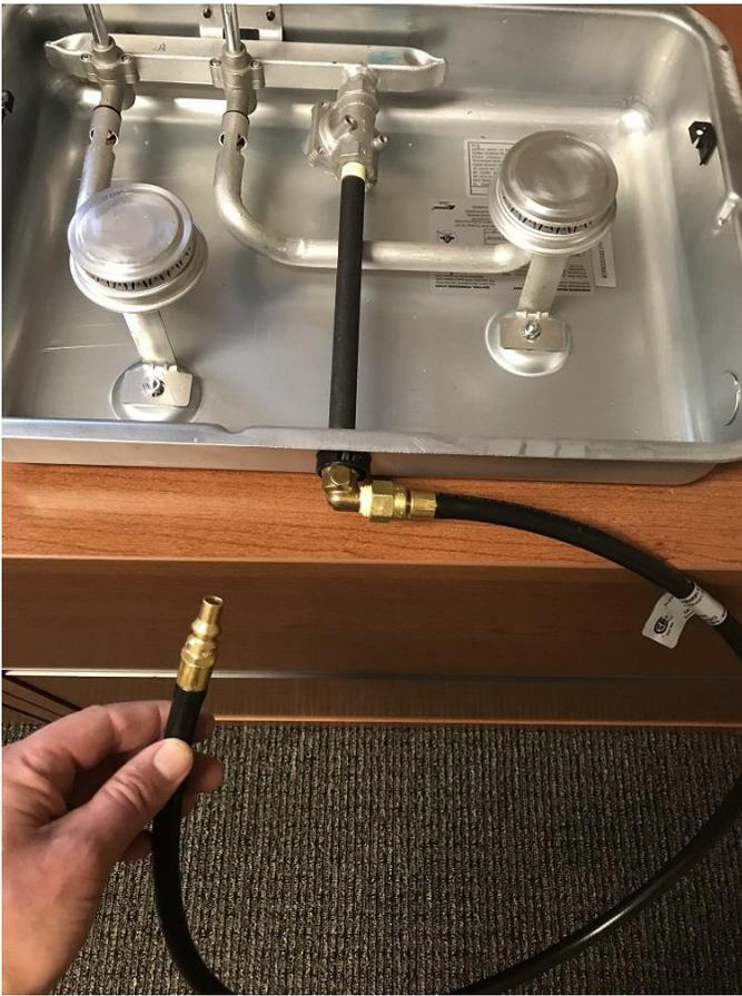
The female portion of the quick disconnect hose can now be attached to the threaded end of the 90 degree elbow, and again wrench tightened.
