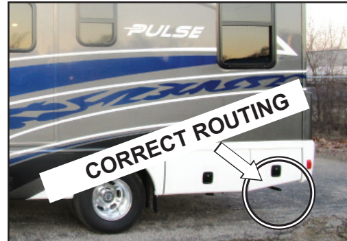
Figure 1 Exhaust pipe is correctly routed as shown located exiting below the rear compartment door latch and extending beyond the sidewall.
