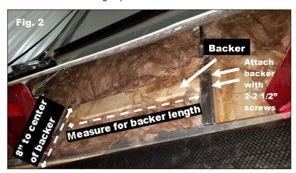
Step 6 Pull the bottom of the skin out and prop open to inspect for wood backer, Figure 2. If backer is present, proceed to Step 8. If there is no backer present, proceed to step 7. **Note:** Pictures of the backer area will be required on the pre-authorization for repair verification.
