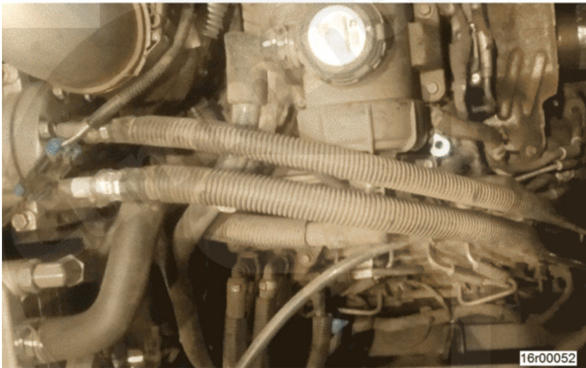
Figure 8, Existing Refrigerant Hose Mounting.
