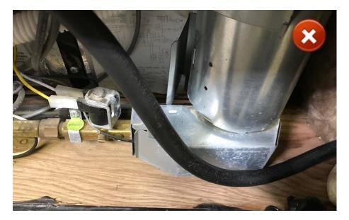
It is critical to have  $\frac{1}{2}$ " minimum / 1" recommended clearance between the LP hose and the burner box.
