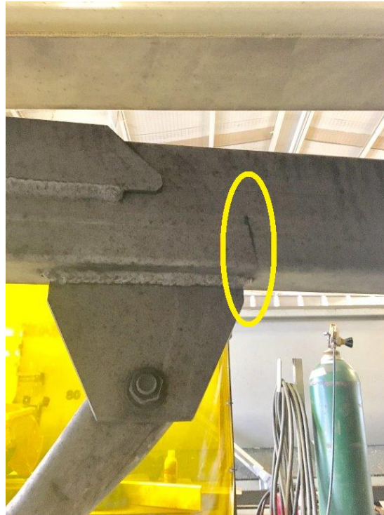
View of crack from inside face of the draft arm tubing
