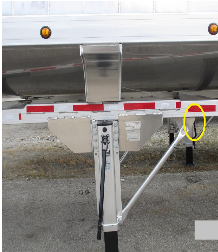
View of area to look for a crack, both sides of trailer
