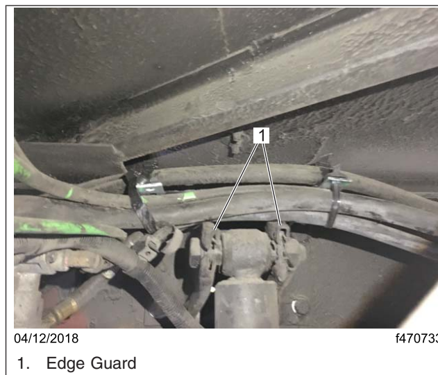
Fig. 17, Inspecting for Edge Guard
