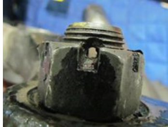
Cotter Pin Hole Position
