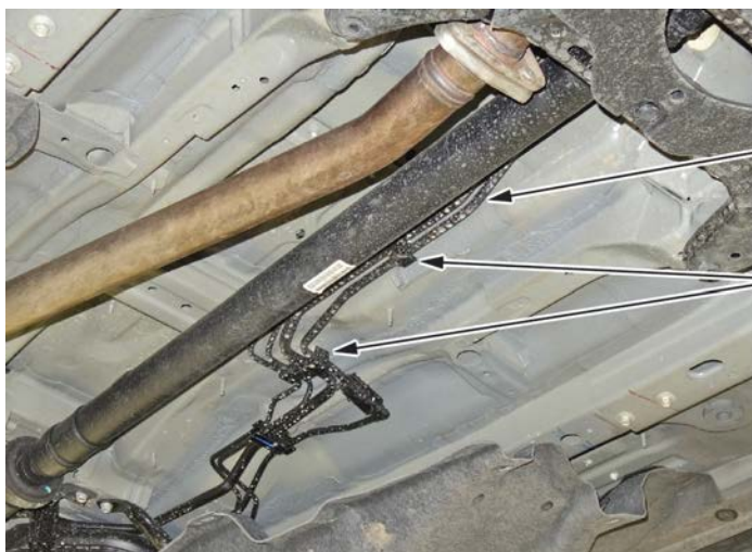
FUEL FEED PIPE Replace.
