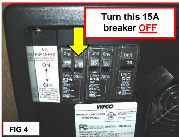
FIG 4: Turn OFF the second breaker (15A) from the left (arrow)
