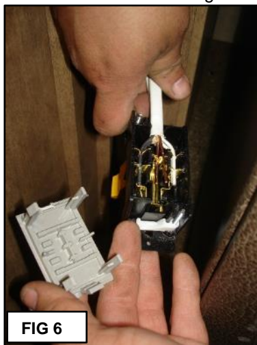
FIG 6: Remove the back of the outlet to expose the wiring.
