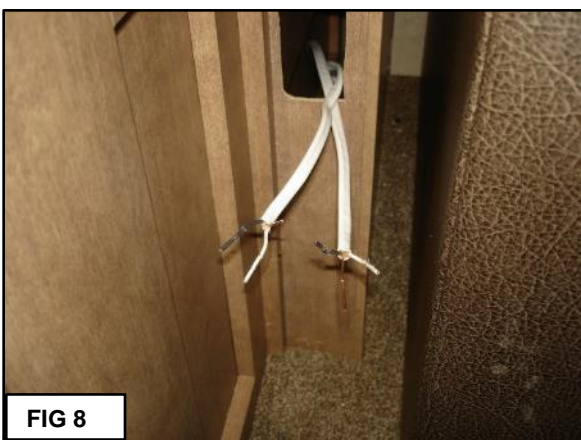
FIG 8: Remove all wires from the outlet.
