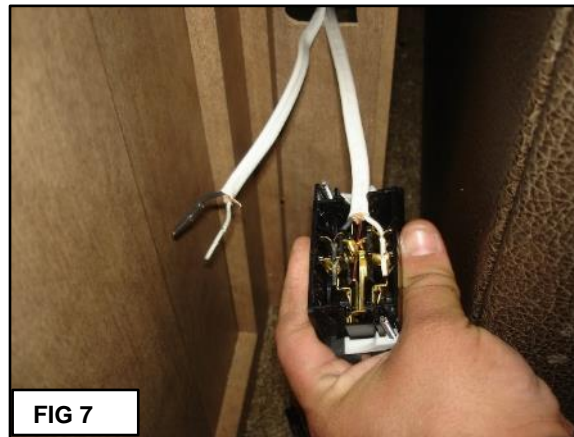
FIG 7: Use the screwdriver to pry the wires from both Romex cables out of the outlet.
