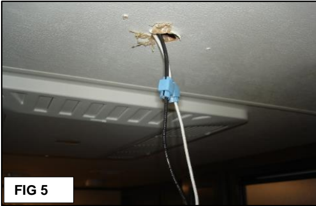
FIG 5: Gently pull the wires down exposing the Scotch lock connectors.
