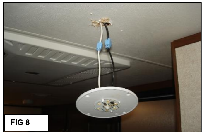
FIG 7: Attach the black and white wires of the new light base to the wires in the ceiling.
