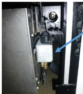
Kneeling Module behind air dryer, curbside.
