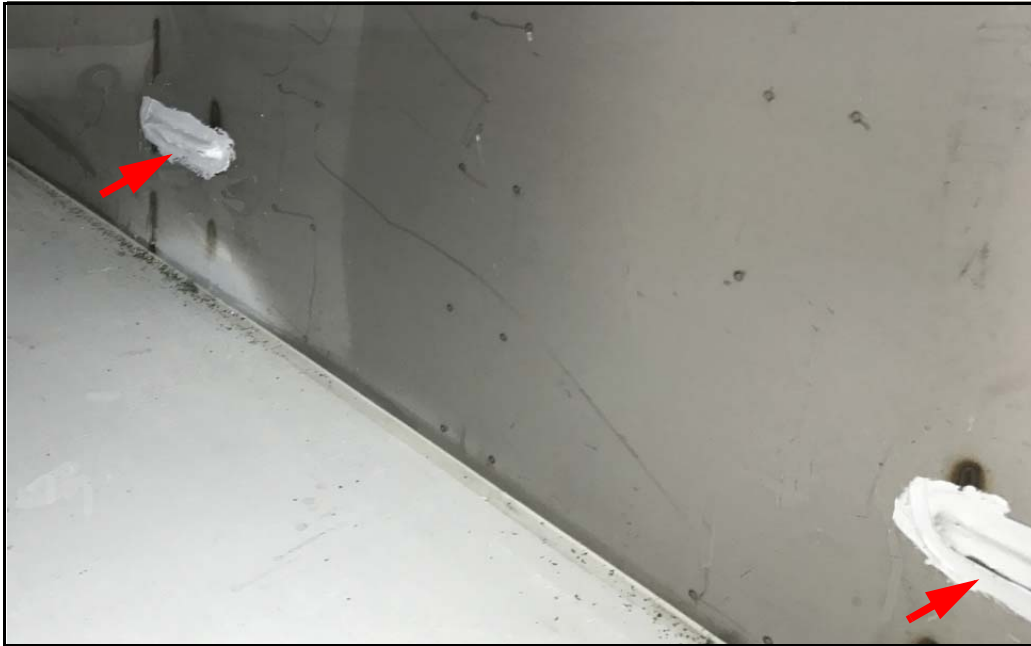
Figure 19. Application of sikaflex to u-bolts and interface area.
