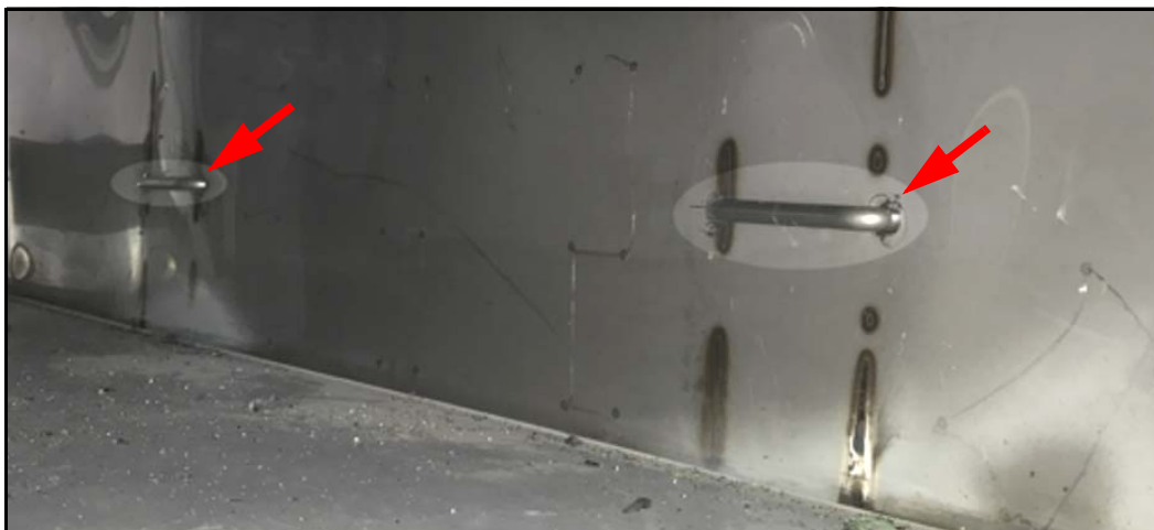
Figure 11. Reference photo of drill holes and u-bolts on front panel of bagg. bay #1.
