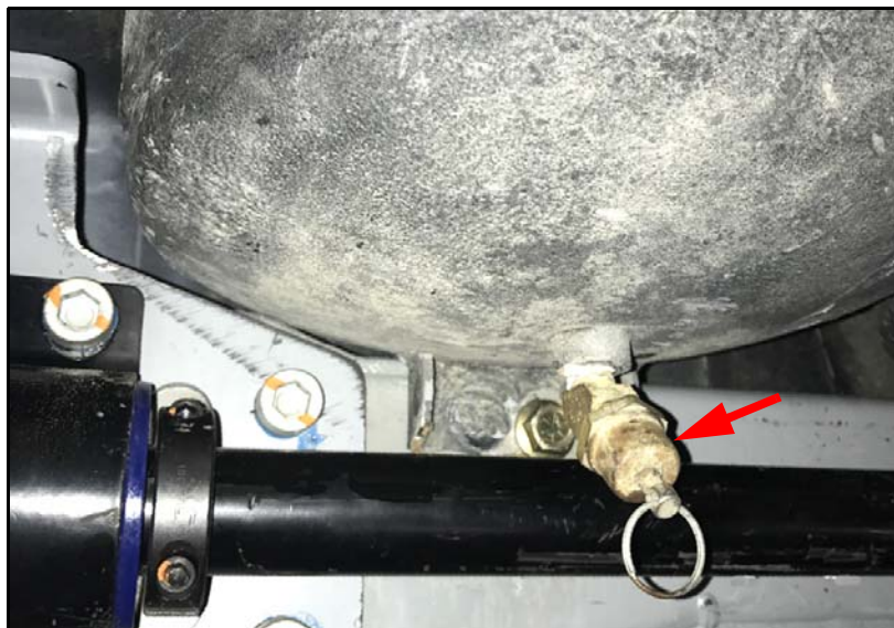
Figure 18. Drain valve installation.
