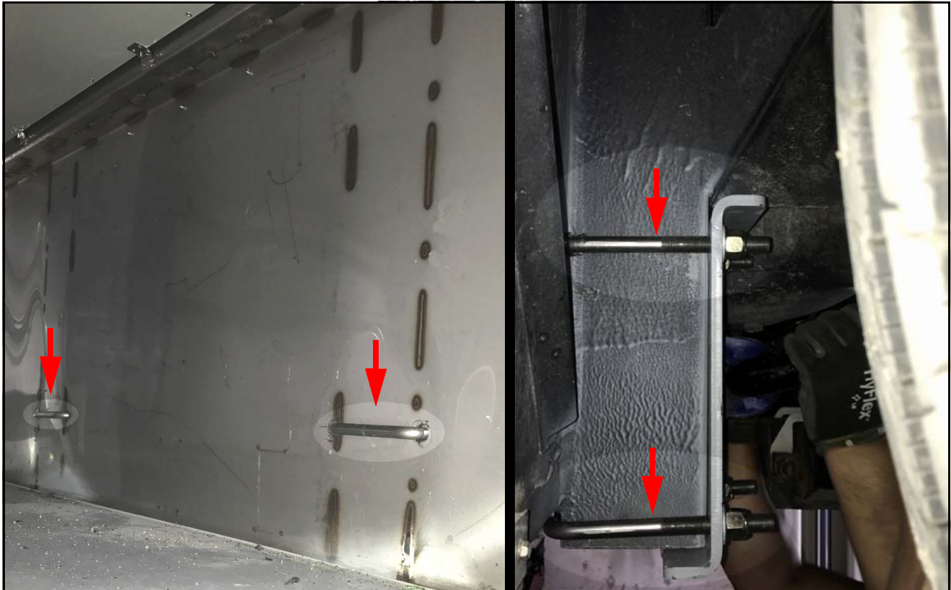
Figure 13. U-bolt routing from the forward bulkhead panel inside baggage bay compartment #1.
