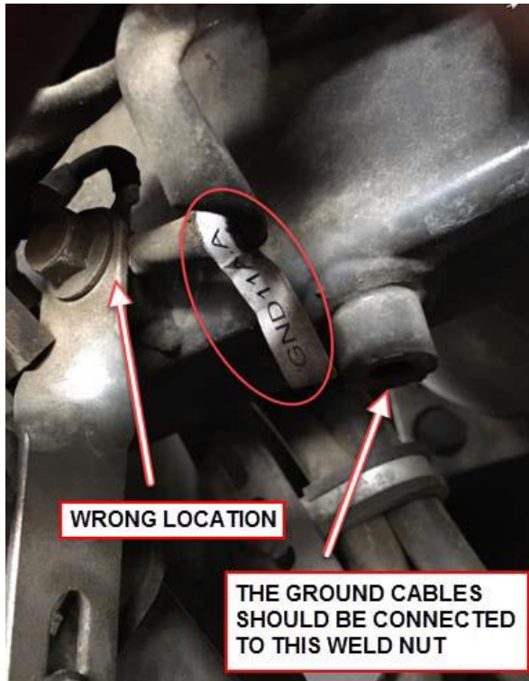
FIGURE 3: WRONG CONNECTION OF GROUND CABLES
