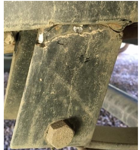
FIG 3: Cracking around the welds/tube
