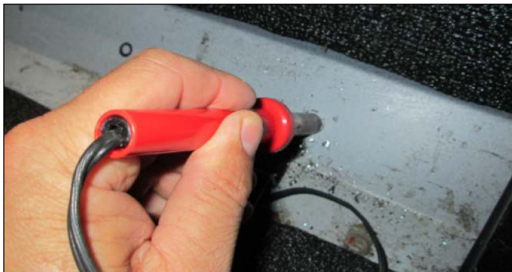
Figure 9: Removing Davenport Insulation
