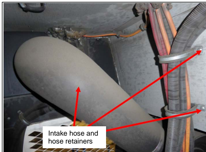
Figure 7: Removal of the Intake hose and hose retainers
