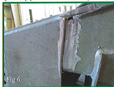
Cracks that are 1/4" or more from top plate weld can be temporarily repaired
