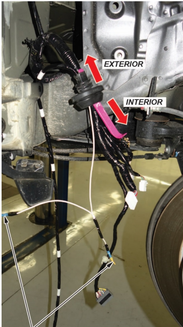
BUTT CONNECTORS ON INTERIOR SIDE
