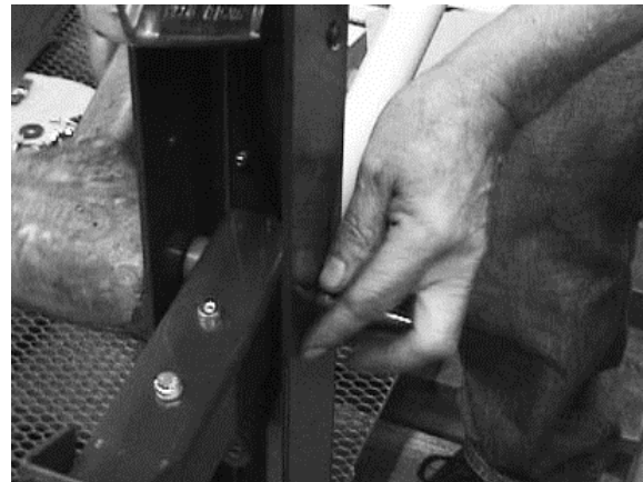
Figure 24. Pin Link Installation
