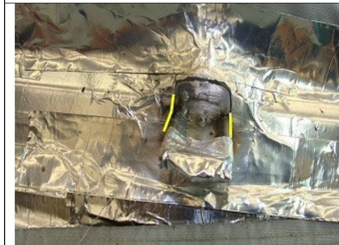
16. Then, weld the right side of the bracket. Continue to weld the right side of the remaining brackets to allow time to cool.
