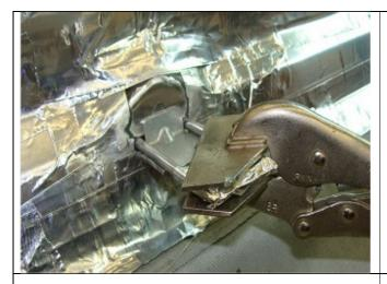
14. Install reinforcement bracket as shown. Secure bracket with suitable clamp.
