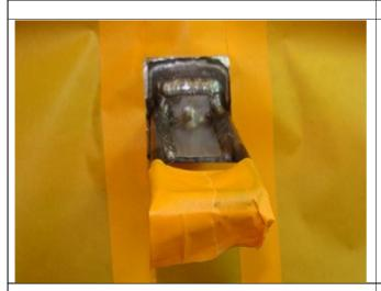
19. Once the welds have sufficiently cooled, prepare the areas to reapply anti-corrosion protection.
