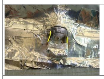
16. Then, weld the right side of the bracket. Continue to weld the right side of the remaining brackets to allow time to cool.
