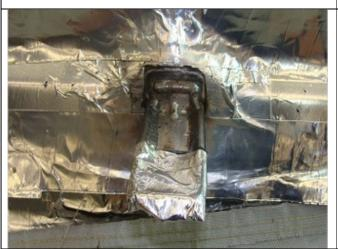
18. Example of properly executed weld is shown. Notice, the welding bead is continuous from left to right side.
