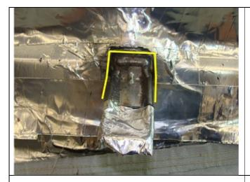
17. Weld a continuous bead of weld to connect the left and the right sides. Complete all remaining brackets in this manner.
