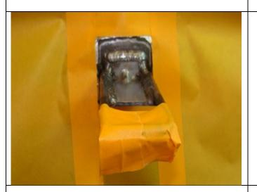
19. Once the welds have sufficiently cooled, prepare the areas to reapply anti-corrosion protection.
