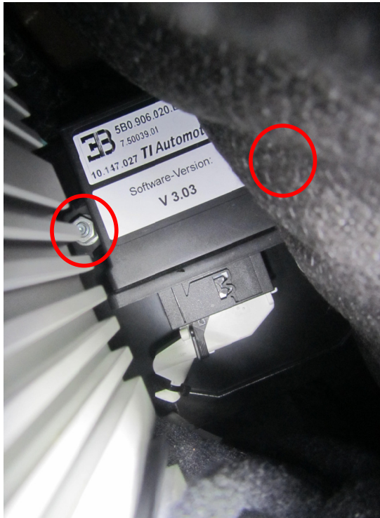
Passenger side view of the Tank Control Unit (while pulling centre rear wall)
