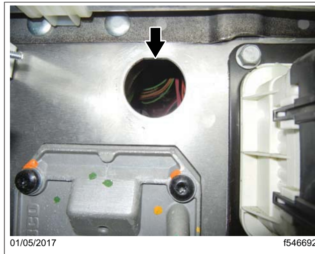
Fig. 32, Bulkhead Connector 1A Cavity on the Frontwall
