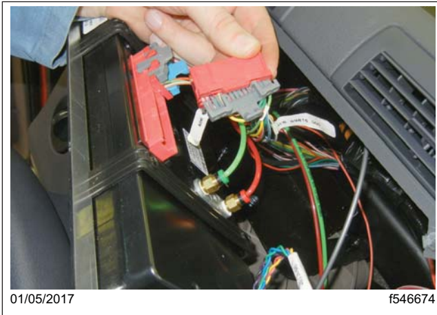
Fig. 14, ICU 2A connector Terminal Locks
