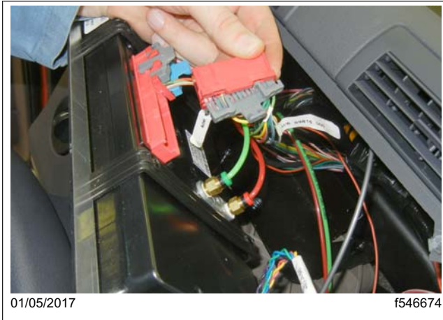
Fig. 15, ICU 2A connector Terminal Locks
