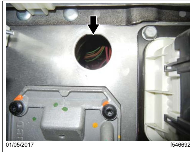
Fig. 32, Cavity of the 1A connector of the partition wall in the front wall
