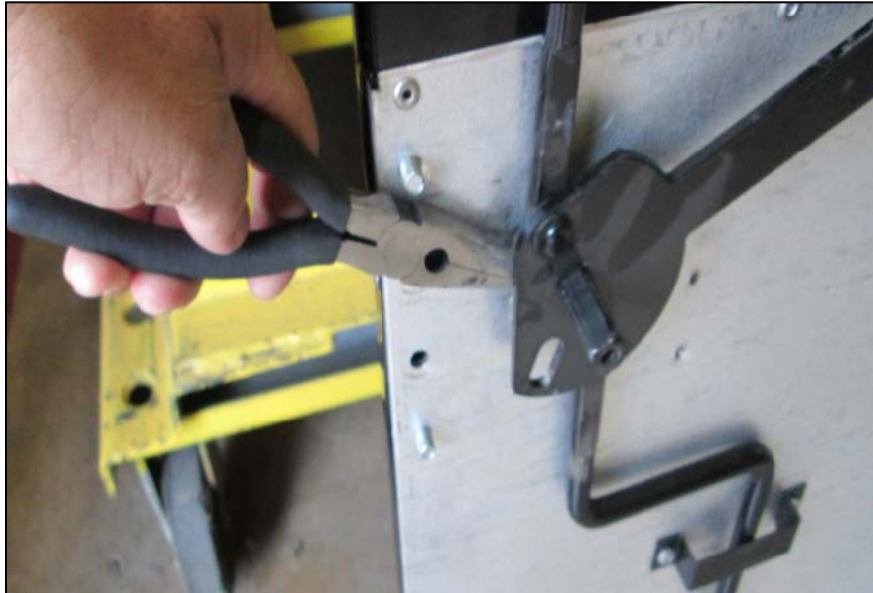
Figure 18, Bending the Roll Pin
