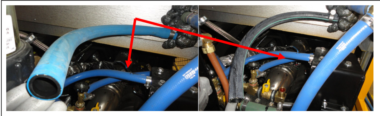
Figure 9, Removal and Replacement of the Supply Line
