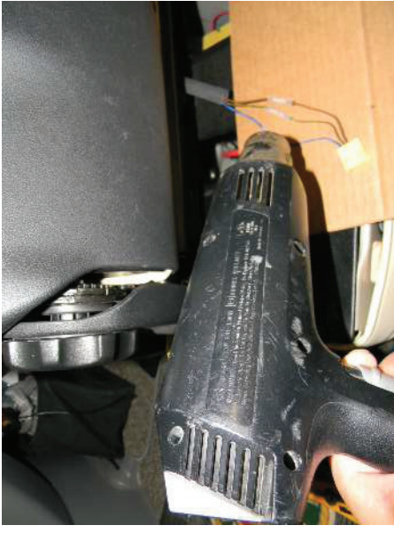
Use heat gun to seal butt connectors and allow connectors to cool before proceeding
