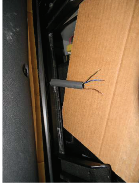
Slide large heat shrink tubing over wires and strip ends
