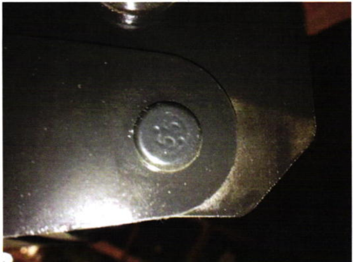
HINGE POINT RIVET MARKED #55 @ 2 nd & 3 rd STEP
