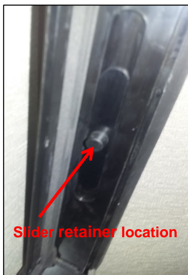
Figure 1, Slide Retainer Installation
