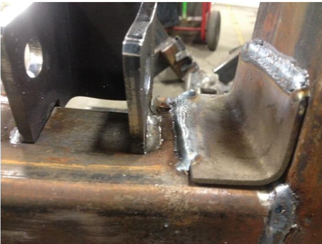
Figure 19: Proposed repair #2 after testing
