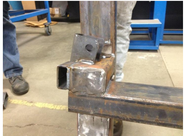
Figure 16: Proposed repair #1 after testing
