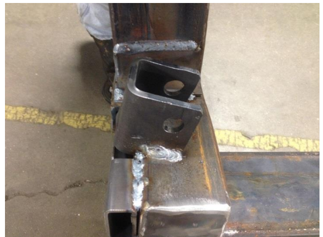
Figure 18: Proposed repair #2 after testing
