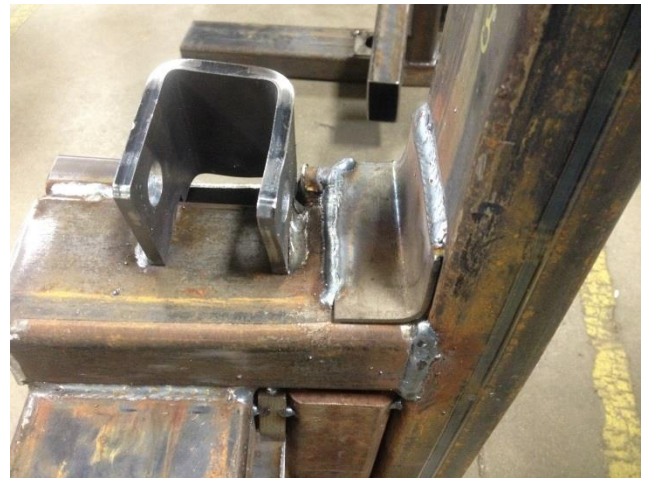
Figure 20: Proposed repair #2 after testing
