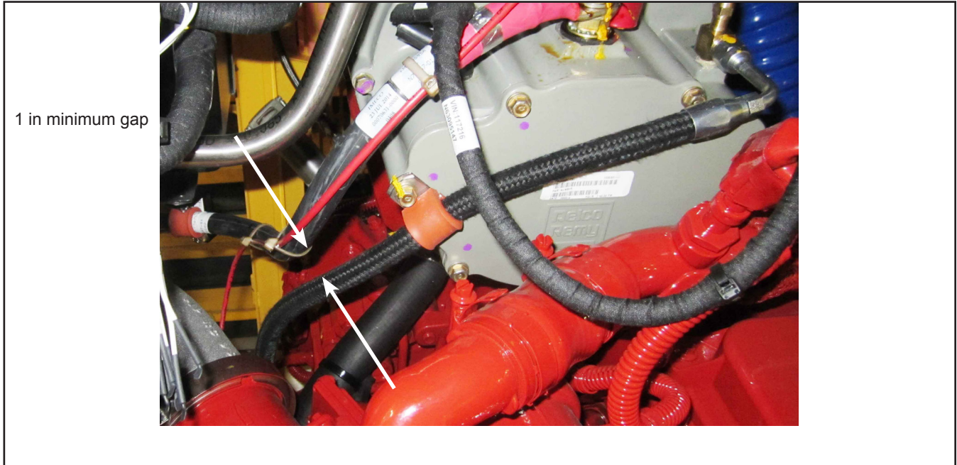
Figure 3 - Flat Terminal Alternator Cable Routing
