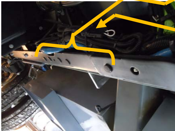
View from underneath
