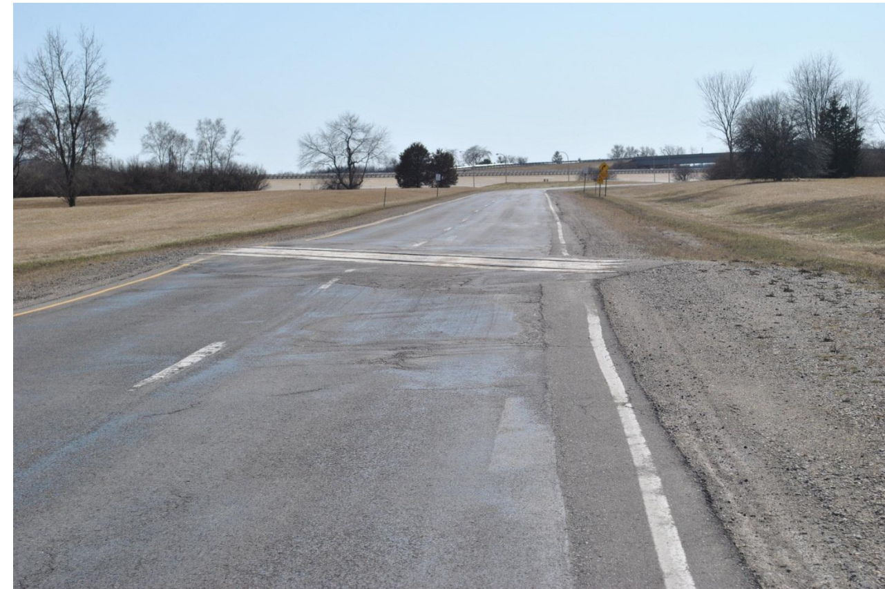
Figure 7b: Ride & Handling Angled RR crossing @ 60 – 80 MPH - An elevated railroad crossing that is not perpendicular to the road direction
