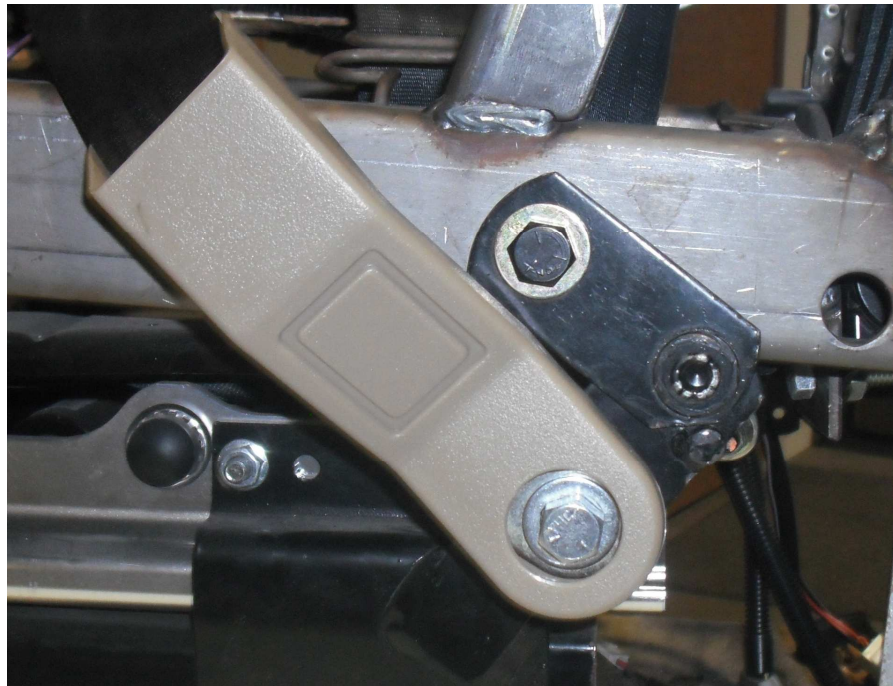
COMPLETED REPAIR TIGHTEN BOLT TO 20 ft-lb
