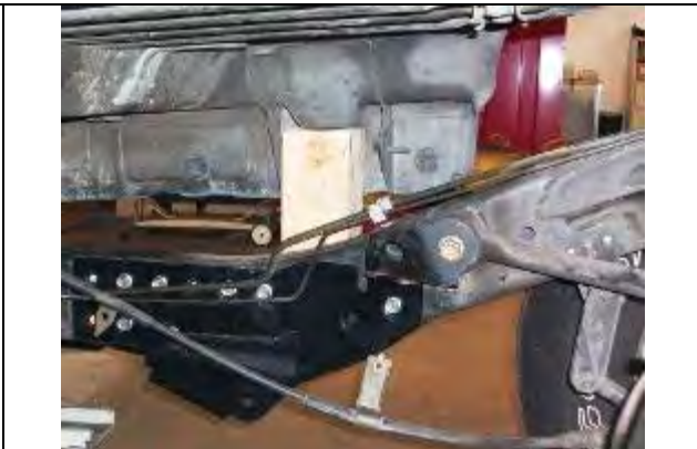
Figure 56 - Wood Block Installed at #4 Body Mount
