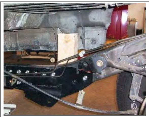
Figure 82 – Wood Block Installed at #3 Body Mount
