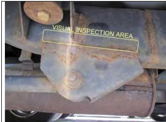
Figure 1 – Visual Inspection Area
