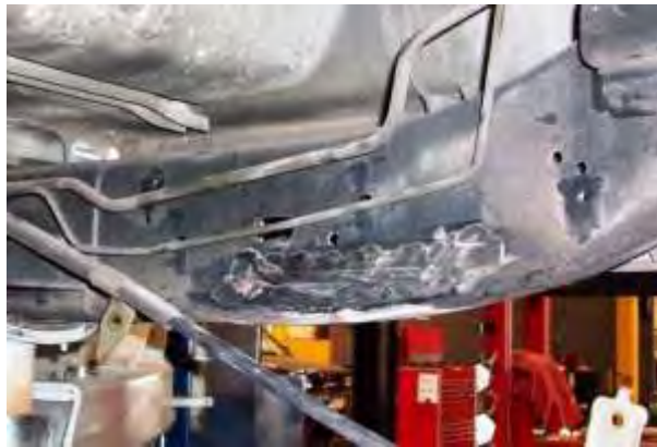
Figure 85 – Frame After Bracket Removal
