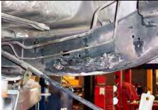
Figure 59 - Frame After Bracket Removal
