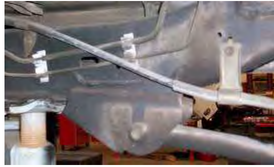
Figure 58 - Passenger Side Bracket Before Removal
