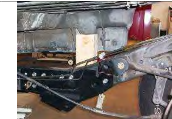
Figure 56 - Wood Block Installed at #4 Body Mount
