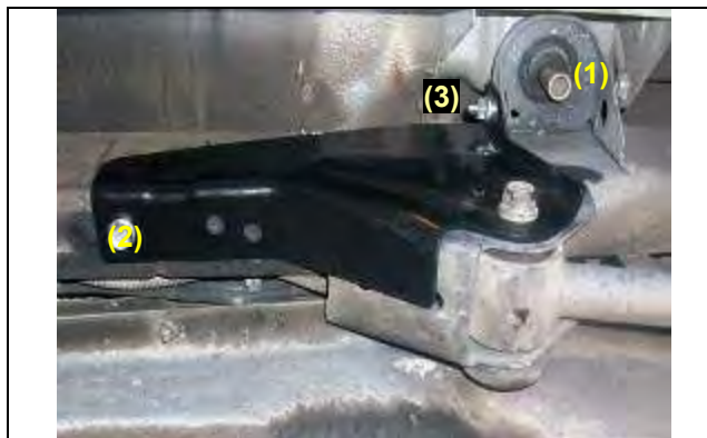
Figure 15 - Driver Side Temporary Installation 1. #4 Body Mount Lower Half Removed 2. Weld Nut Already in Frame 3. Stud and Nut
