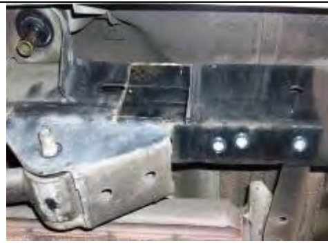
Figure 22 - Passenger Side Pop-nuts Installed
