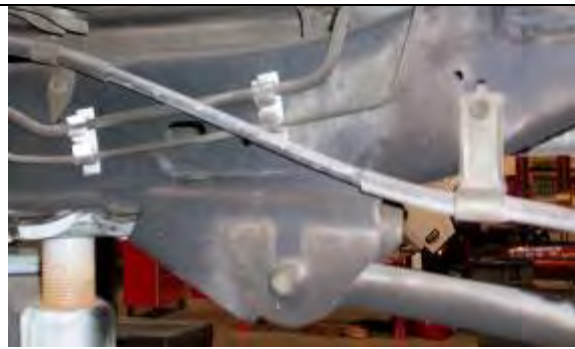
Figure 84 – Passenger Side Bracket Before Removal
