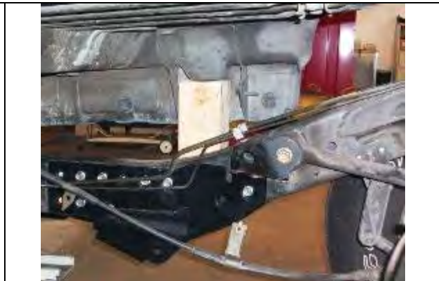
Figure 56 - Wood Block Installed at #4 Body Mount
