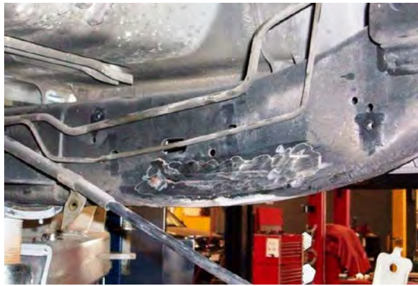
Figure 85 – Frame After Bracket Removal
