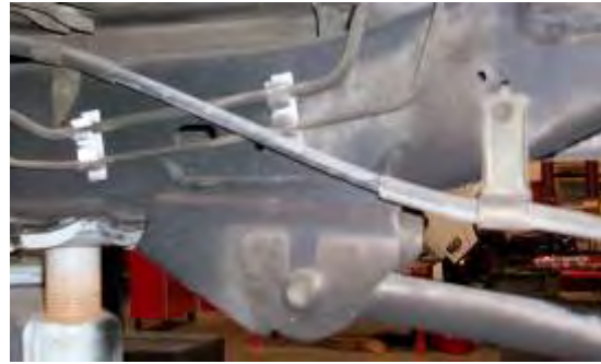
Figure 58 - Passenger Side Bracket Before Removal
