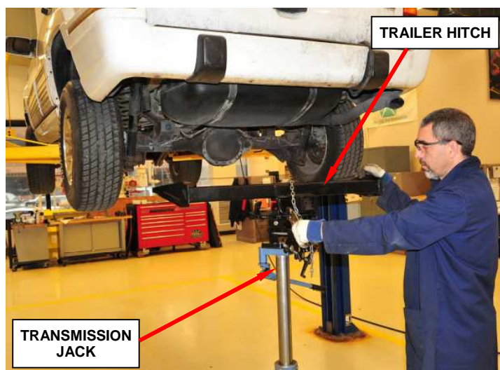
Figure 9 – Install Trailer Hitch into Position
