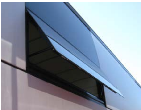
Fig.1 Typical awning-type window
