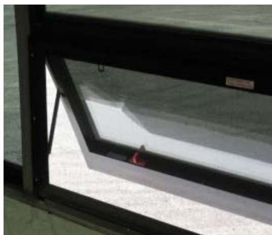
Fig.2 Inside view of an awning window
